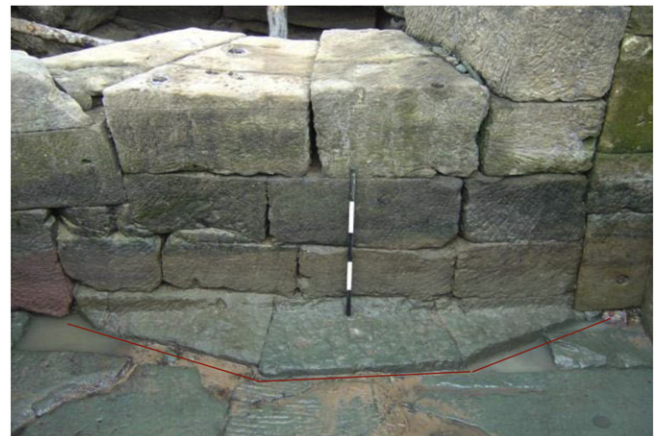
Fig. 18. Overlapping structure of the Western wall of the Eastern shaft (Fletcher).
