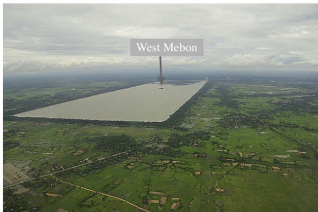
Fig. 4. The vast West Baray with the West Mebon at its center—view from the west (Evans).
